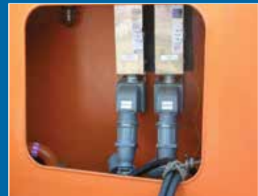
200A MaxGard® inlets with disconnects
