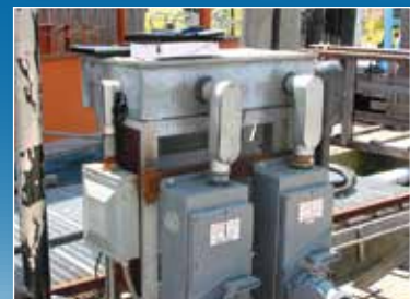
200A MaxGard® interlocks in parallel
