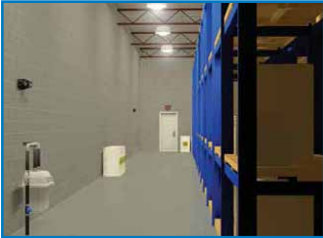
3D image showing installation of two NXM Series battery units and a ENC combination unit in an industrial application under normal lighting conditions.
