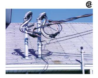
01 MM801, heavy-duty 400 A spool rack — 02 MM806N, 4 inch neoprene roof flange — 03 CIEFA-4, 4 inch entrance head —
