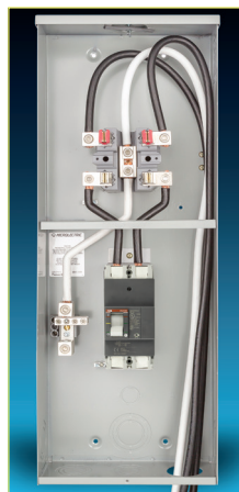
Step 2 Install line side conductors.
