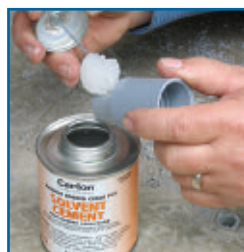
Apply a uniform coat of cement.
