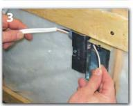
Insert the cable into the box.
