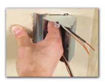
The innovative design will allow you to easily extract the box without damaging the drywall.
