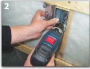
Screw the box to the stud using the center hole for one screw mounting.
