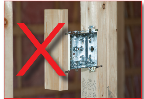
This installation does NOT COMPLY with C.E.C. 12-3010 (3).
