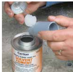
Apply a uniform coat of cement.
